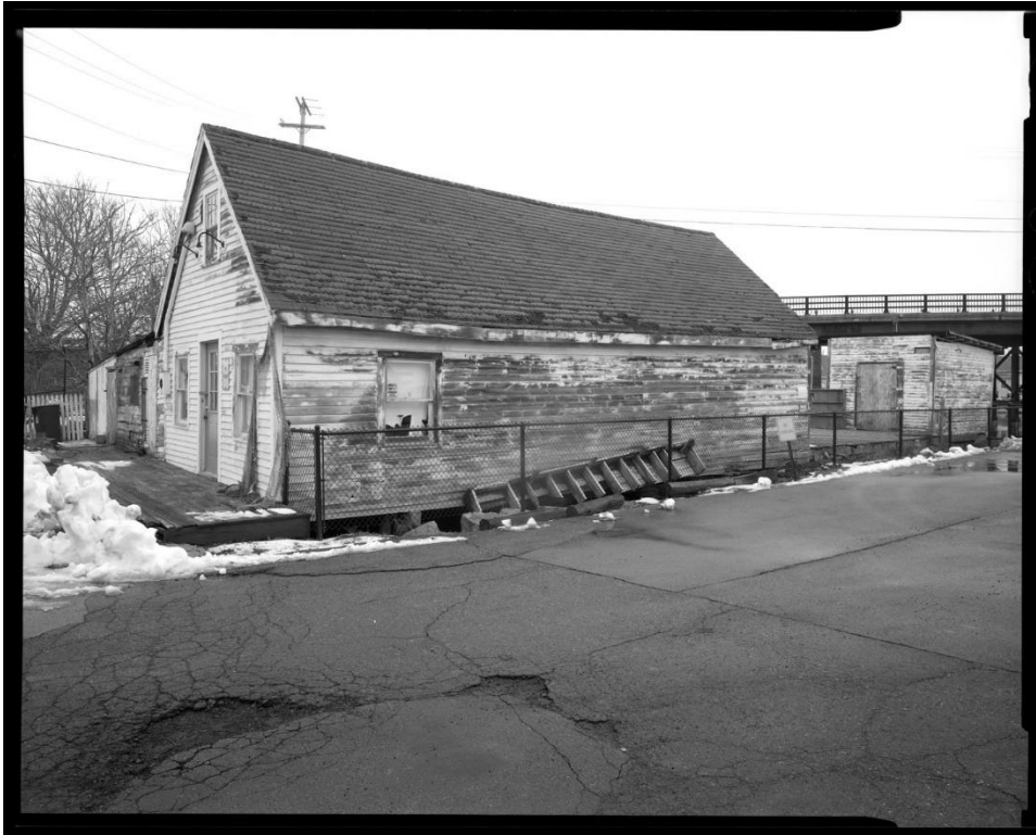
NH-566-7: South elevation of Market, Office & Shop (A) and west and south elevations of South Storage Shed (C). Looking northeast.
