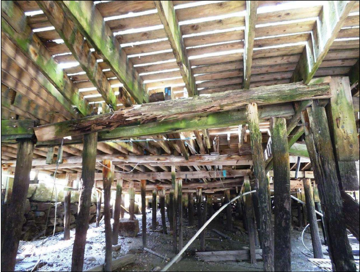
FIGURE 6: Photo of underside of wharf taken at low tide showing wood pilings and posts supporting deck and buildings above. Granite retaining wall of solid City Pier seen at left. (Source: Waterfront Engineers LLC, 2014).
