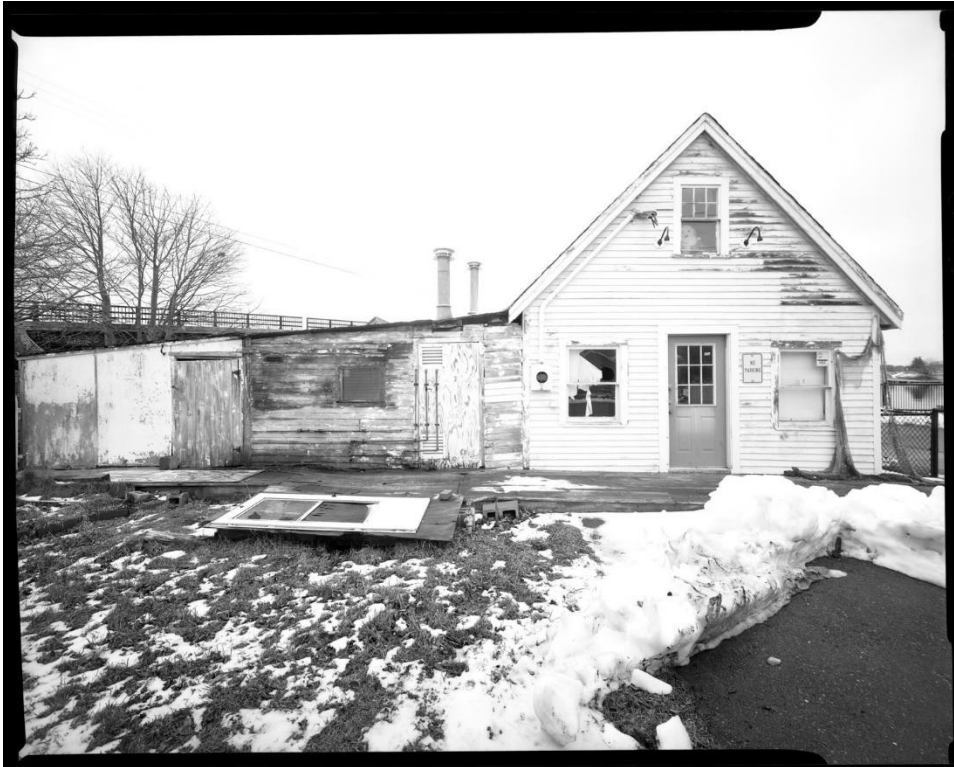
NH-566-6: Front (west) elevation of Market, Office & Shop (A), showing shed-roof additions to left, Lobster Pound (A-1) and Storeroom (A-2). Looking east.
