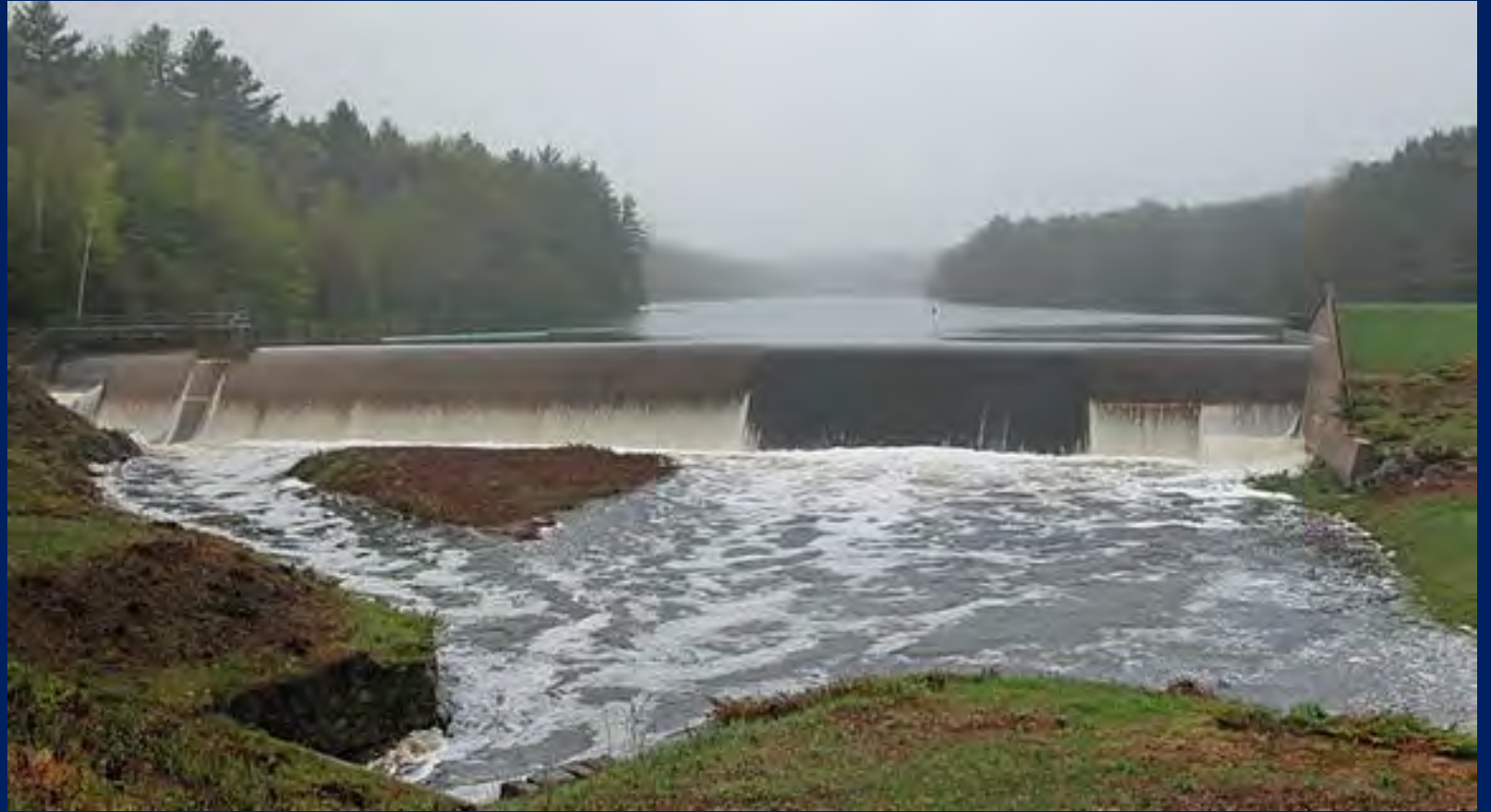
Bellamy Dam "Mother's Day Flood" 2006
