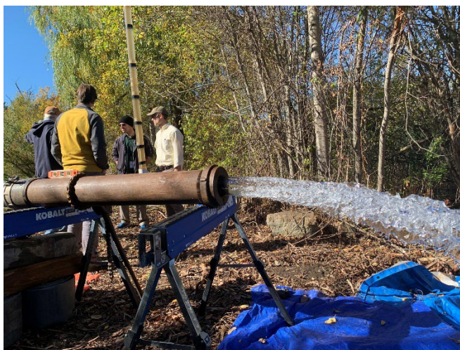
Pump Testing Collins Well 2 – October 2022
