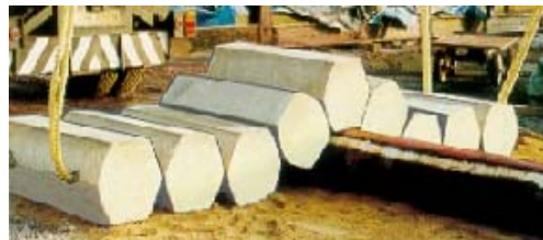
4m x 1.5m x 450mm Mattress draped over a 20" pipe.
