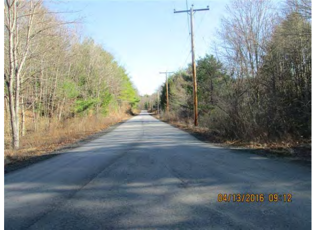
Figure 2-8: Paved Roadway #2, MNTM on right side EOP
