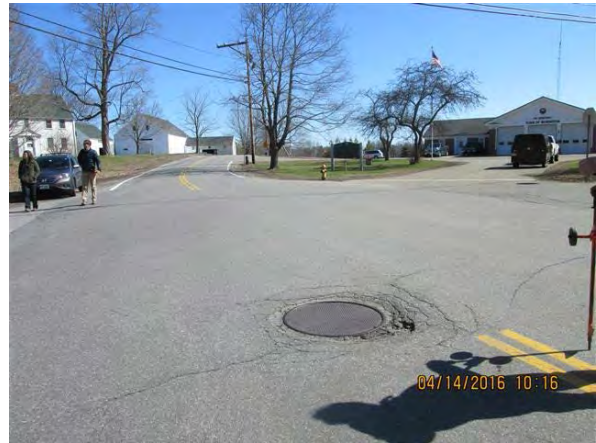
Figure 2-75: 24" GV chamber at Nimble Hill Road and Fox Point Rd.
