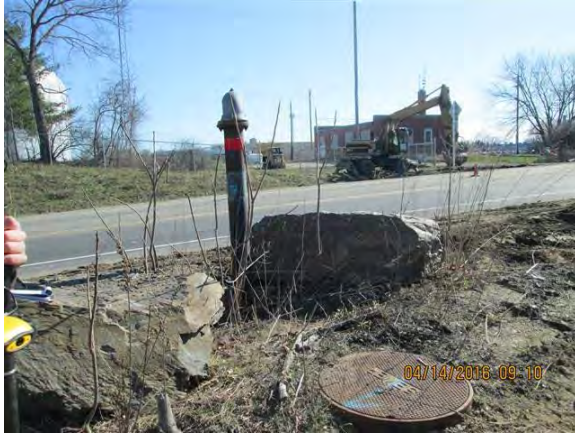
Figure 2-72: 2" Air Release Valve, chamber and vent, #21 near Newington BPS
