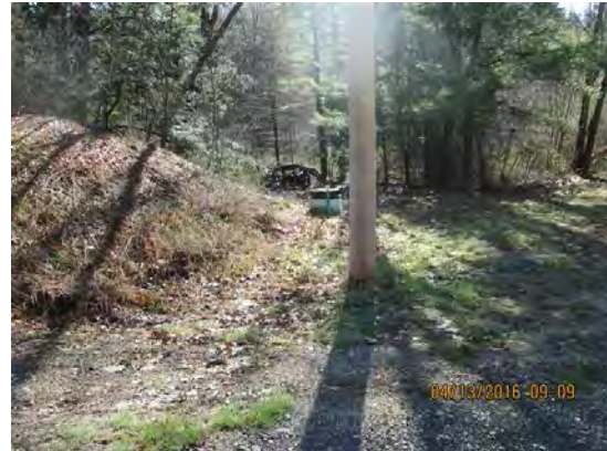
Figure 2-4: 1" service near Well Station #3
