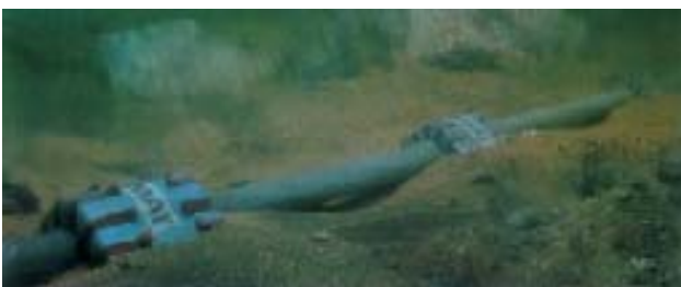
Prevention of pipelift and snaking.
