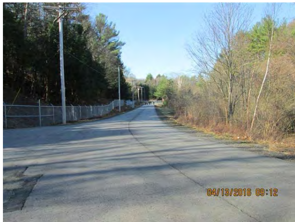
Figure 2-9: Paved Roadway looking toward Well Station #1
