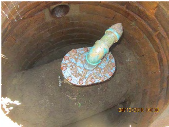
Figure 2-17: 2-inch Air/Vacuum Valve in Horse farm
