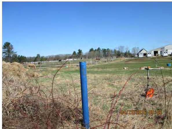
Figure 2-18: Pipe marker assumed to be at 8-inch pipe and service connection in Horse farm property
