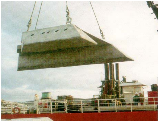
Impact resistant covers (trawlboard and dropped object) for expansion spools on the TOTAL Dunbar Project.
