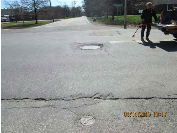
Figure 2-76: 24" Gate Valve in concrete chamber at Nimble Hill Rd and Fox Point Rd.
