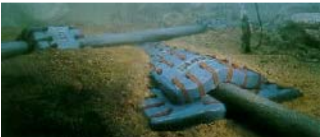
Stabilisation and separation padding for pipeline crossovers.
