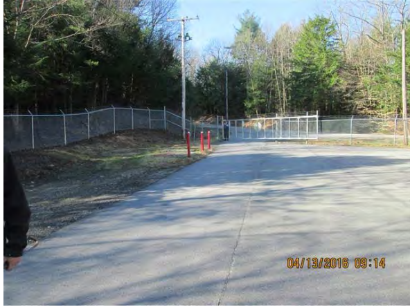
Figure 2-11: Access Gate to Freshet Road near Well Station #1
