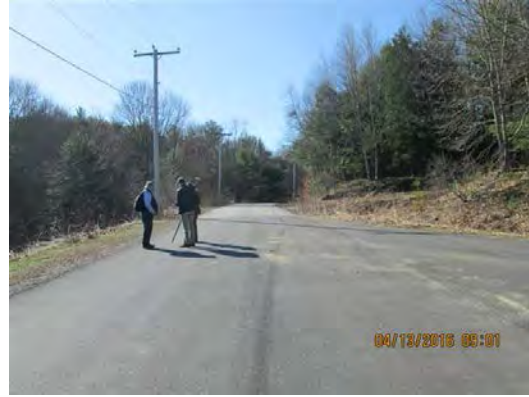
Figure 2-2: MNTM installed on left side of paved road
