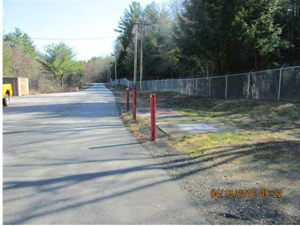
Figure 2-15: Looking up access road toward Well #2
