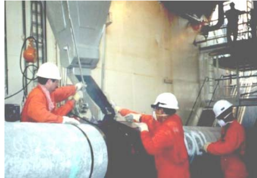
Hot Pouring of Granular Marine Mastic
