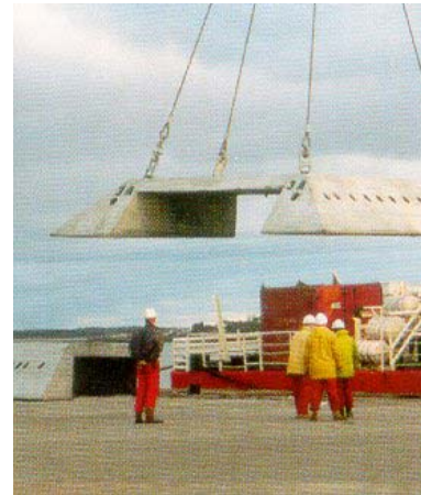
Impact resistant covers (trawlboard and dropped object) for expansion spools on the TOTAL Dunbar Project.
