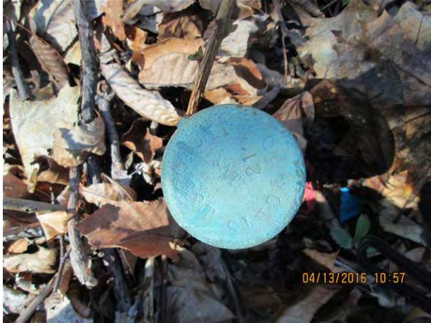
Figure 2-35: Numbered Pipe Markers found at various locations
