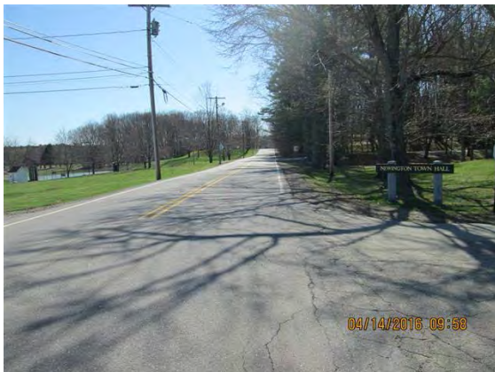
Figure 2-78: Looking south on Fox Point Rd. along MNTM
