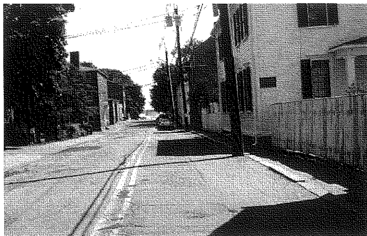
4.2 Court Street in Portsmouth, N.H., showing the path of the 1813 fire. Buildings on the right are part of Strawberry Banke Museum and of eighteenth- or early nineteenth-century date. Those on the left are all post-fire structures.
