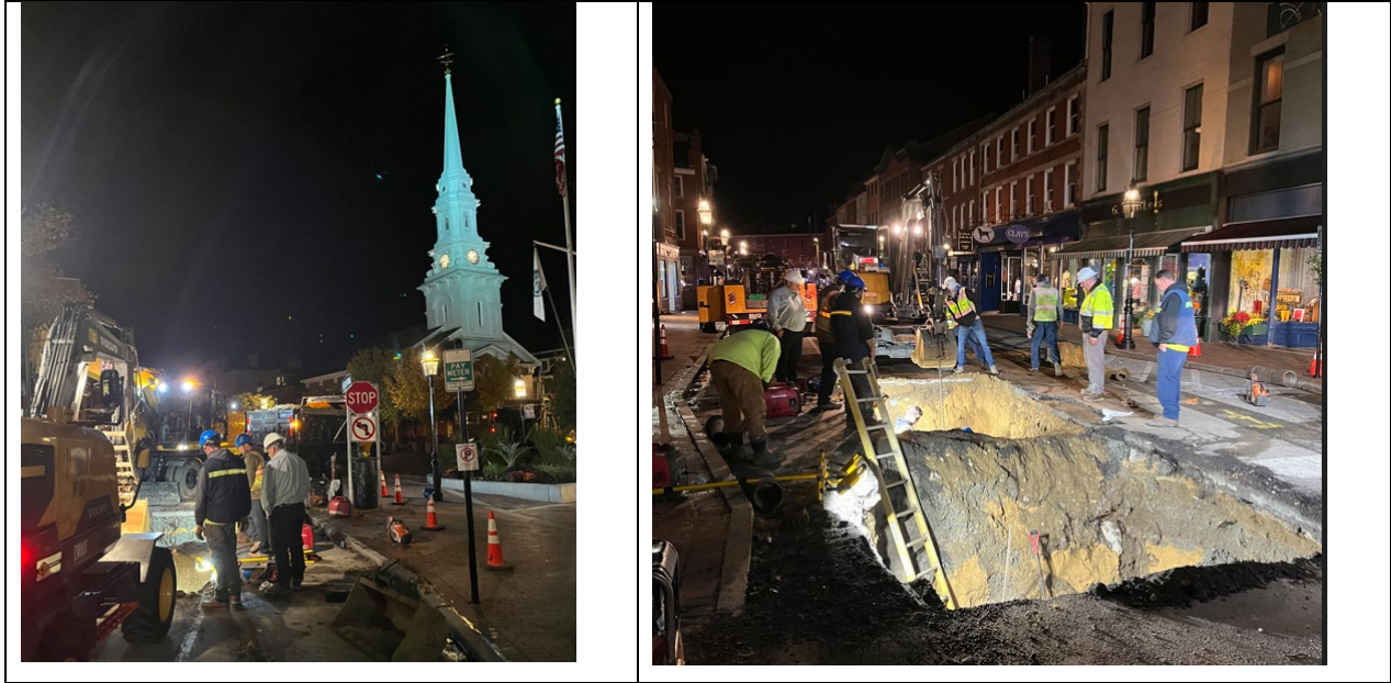
Market Square Water Valve Replacement Project 2:37 AM – October 13, 2023
