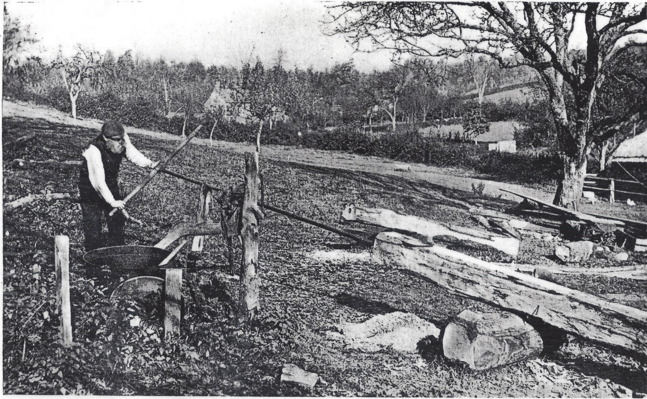
61 Boring elm water-pump pipes by hand, using an auger supported on a rest; Lugwardine, Herefordshire, about 1900
