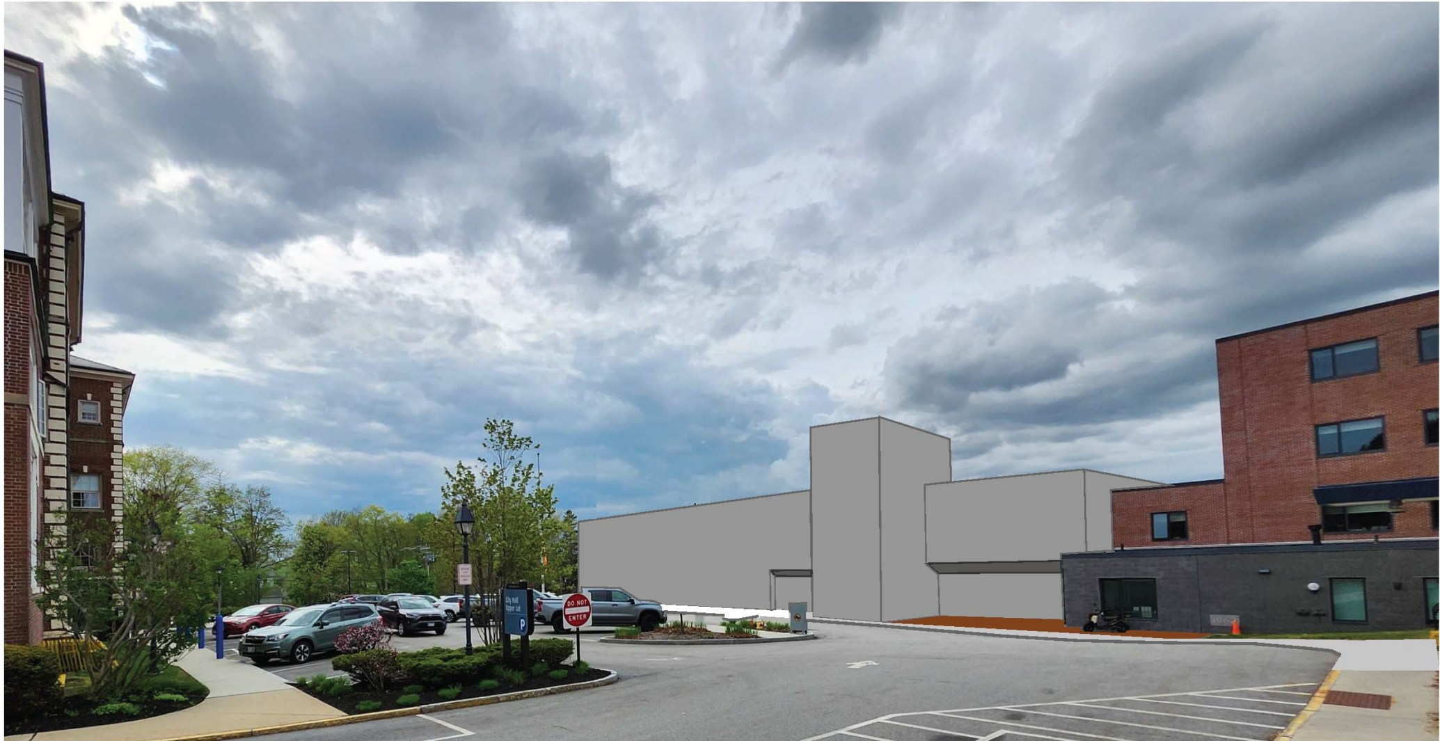
ENTRY VIEW FROM PARKING
