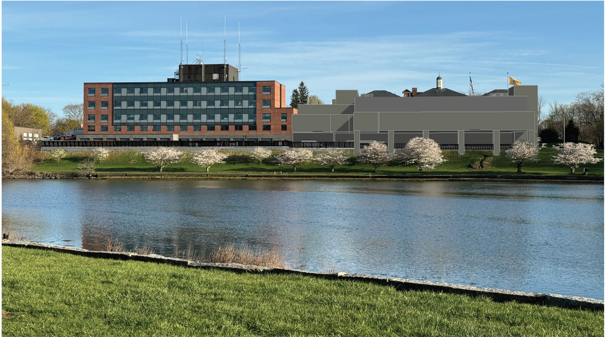
VIEW ACROSS THE MILL POND
