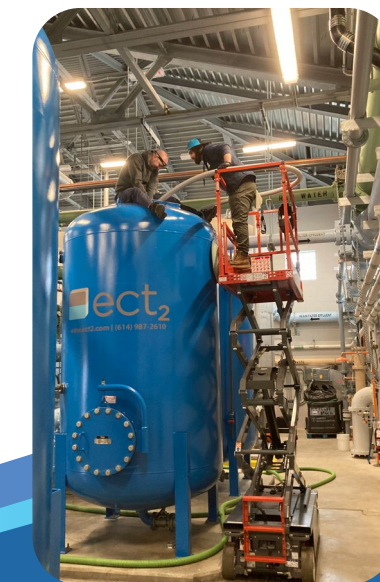
Loading of new ion-exchange resin media into existing vessels.
