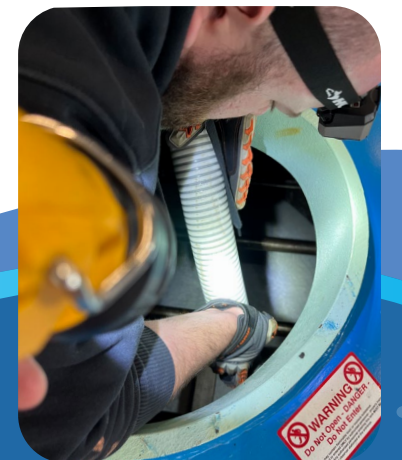
Loading of new ion-exchange resin media into existing vessels.
