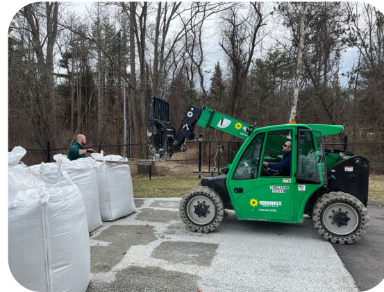
Pease Water Treatment Operators removing bags of spent ion-exchange resin to prepare for new media.
