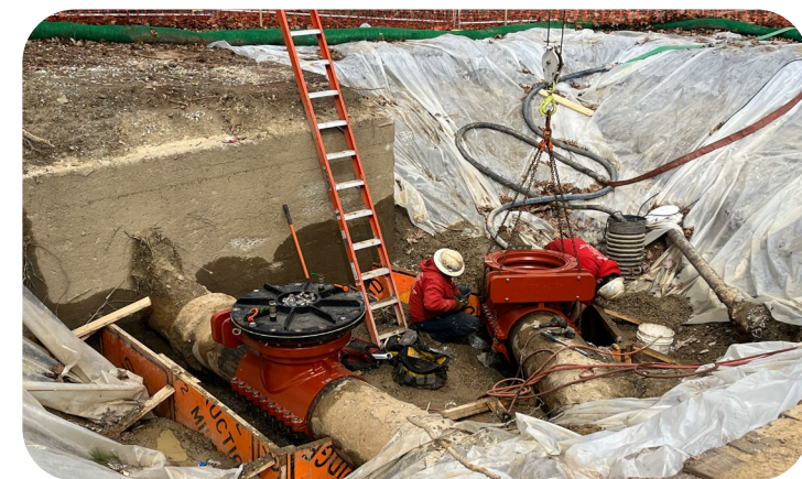
Little Bay water line valve replacements.
