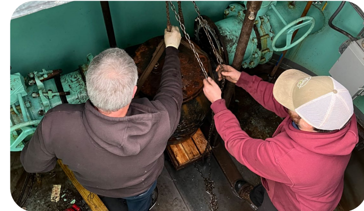
Spinney Tank valve replacement.
