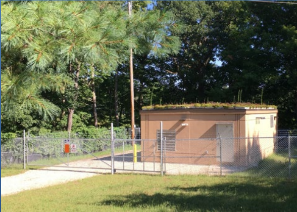
Greenland Well Replacement and New Pumphouse 2018 648,000 Gallons-per-Day
