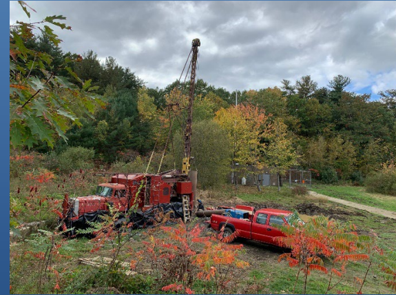
Collins Well 2 Drilled in 2021 (ongoing)
