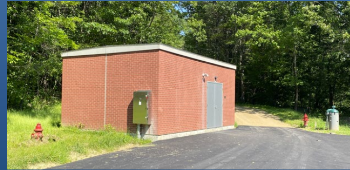
New Pumphouse for Well 4R and 5
