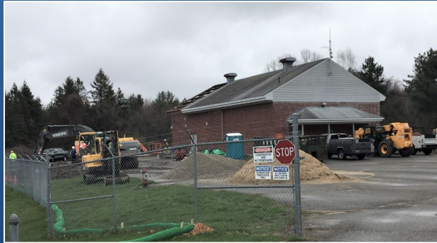
April 2019 – Construction of New Treatment Begins
